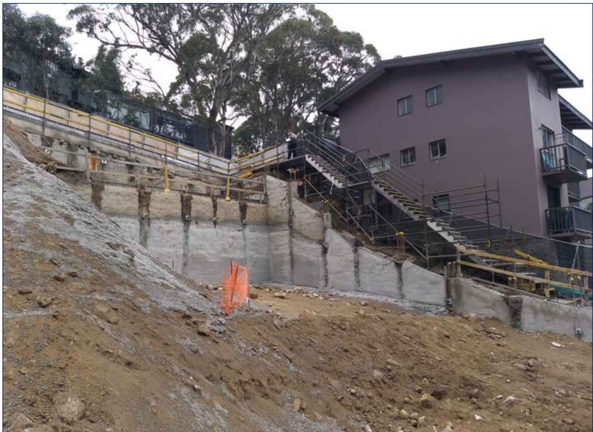
Figure 2 | Existing site excavation and installation of retention structures (Source: Department inspection)
